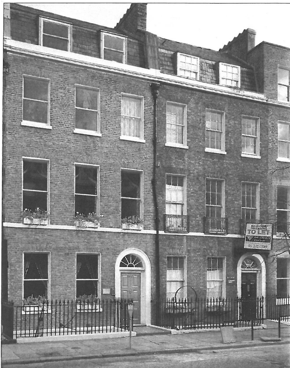
BELOW: Doughty Street, London. Listed buildings in use as professional offices.
